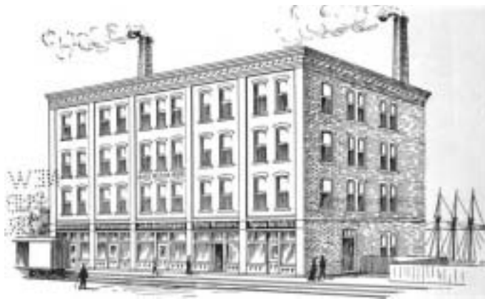
The Bird Block on Sea Street (Tillson Ave). Built in 1898, wholesaler in groceries and manufacturer of the "Three Crow Brand". Now the home of the US Coast Guard in Rockland.
